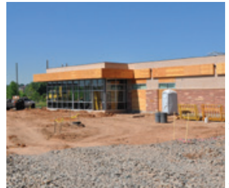
Horticultural Center nearing completion
