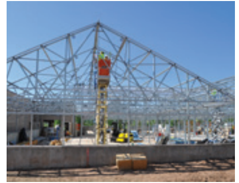
Greenhouse under construction
